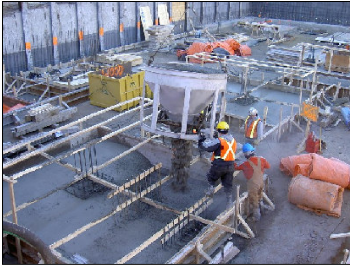
Figure 11: Pad Footing Pour in January at Courtyard on Bear
