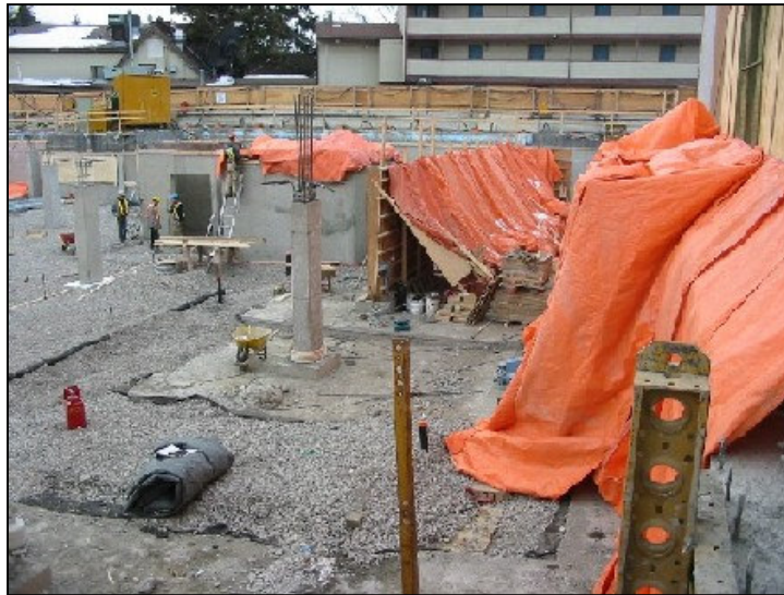
Figure 4: Insulated tarps and heaters enclosing recent wall pours
