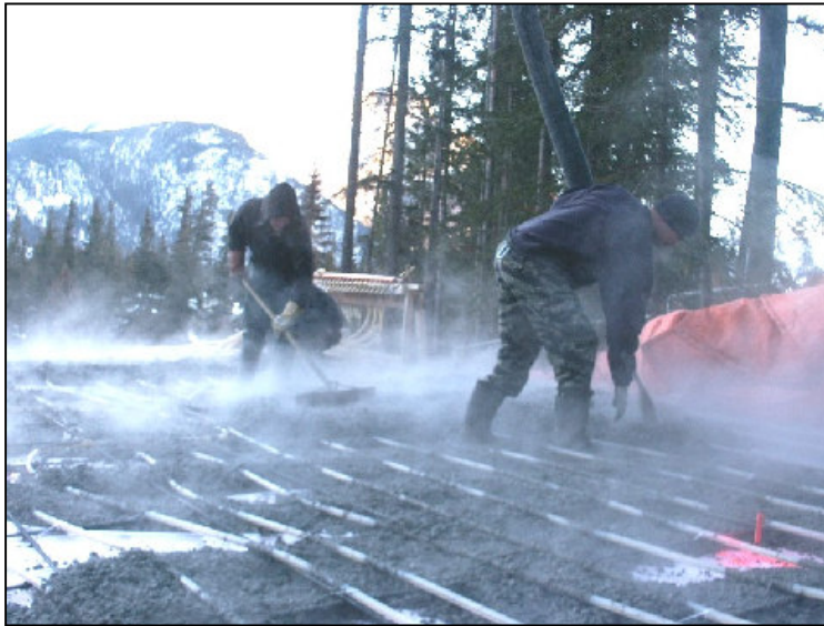
Figure 17: Pouring a slab at Cave Avenue at -25°C
