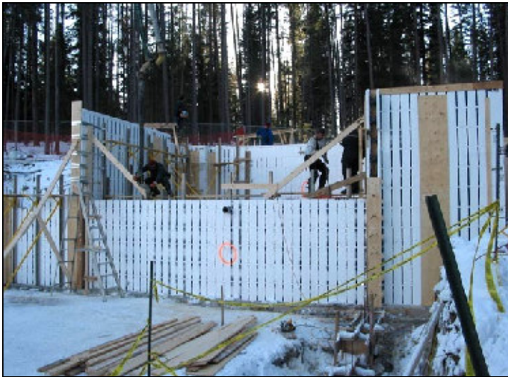
Figure 15: ICF Foundation Walls at Cave Avenue Housing
