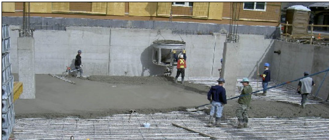
Figure 7: 25% fly ash slab-on-grade pour at Courtyard on Bear
