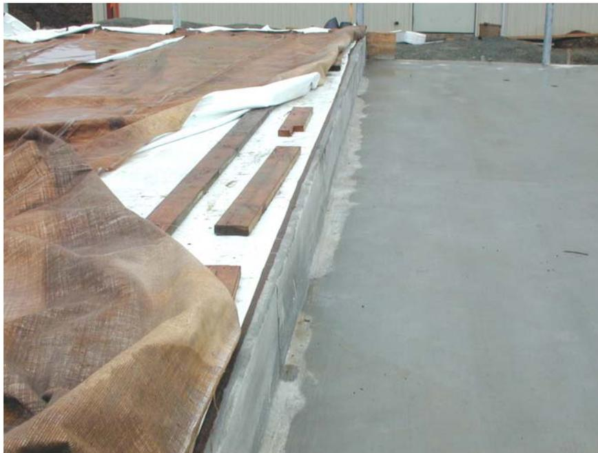
**Figure 5: Moist curing of EcoSmart concrete slab**
