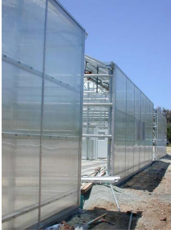
**Figure 3: Greenhouses with Polycarbonate Panels**
