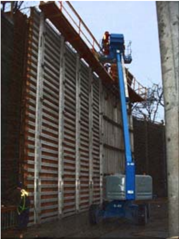
Photograph 3 Wall forming system. Installing thermocouples and maturity gauges.
