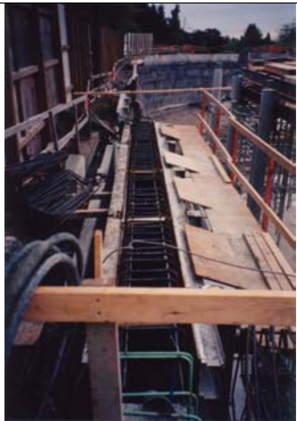
Photograph 12 Top of Wall. Wire in foreground is for thermocouples.
