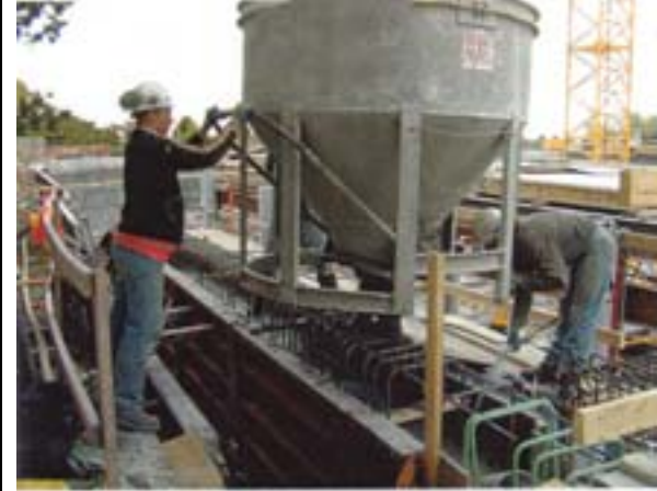
Photograph 13 Placing and vibrating concrete.
