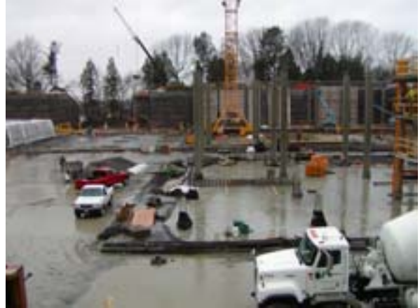
Photograph 2 Phase I Test Wall is one with forms to right.
