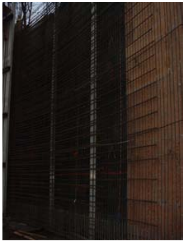
Photograph 4 Wall reinforcement.
