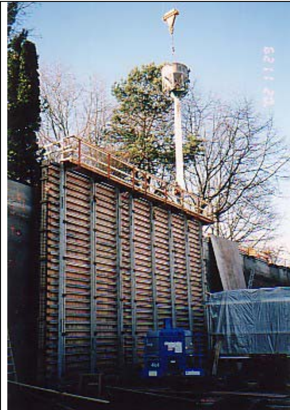
Photograph 5 Phase I. Concrete Placement in Wall.
