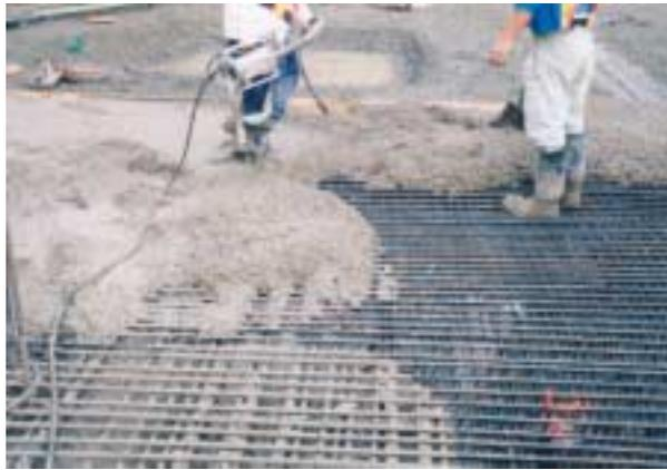
**Fig.4. EcoSmart Concrete- Placing & Vibration (Floor)**
