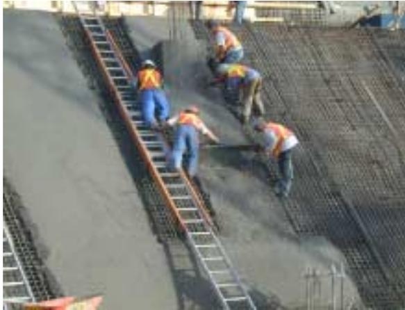
**Fig.3. Applying Structural Shotcrete on Sloping Rock Face**
