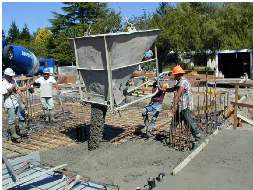
Figure 5: Pouring First Slab with Concrete Bucket
