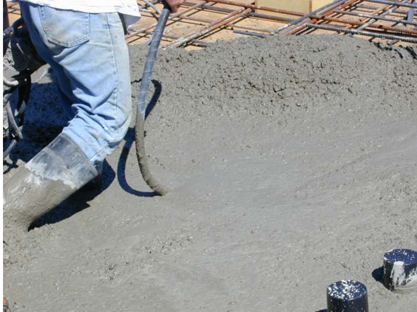
Figure 6: Close-up during Vibration
