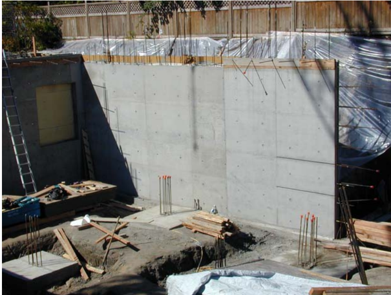
Figure 1: Initial Test Wall Showing 3 Plywood Surfaces
