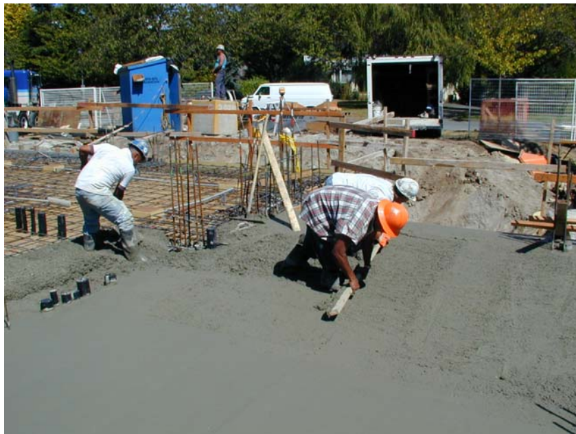
Figure 7: Screeding the Concrete
