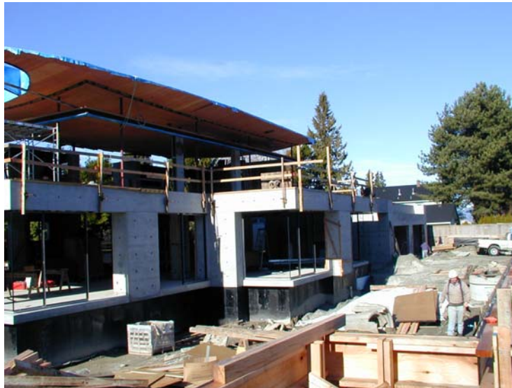
Figure B-2: View of East Walls
