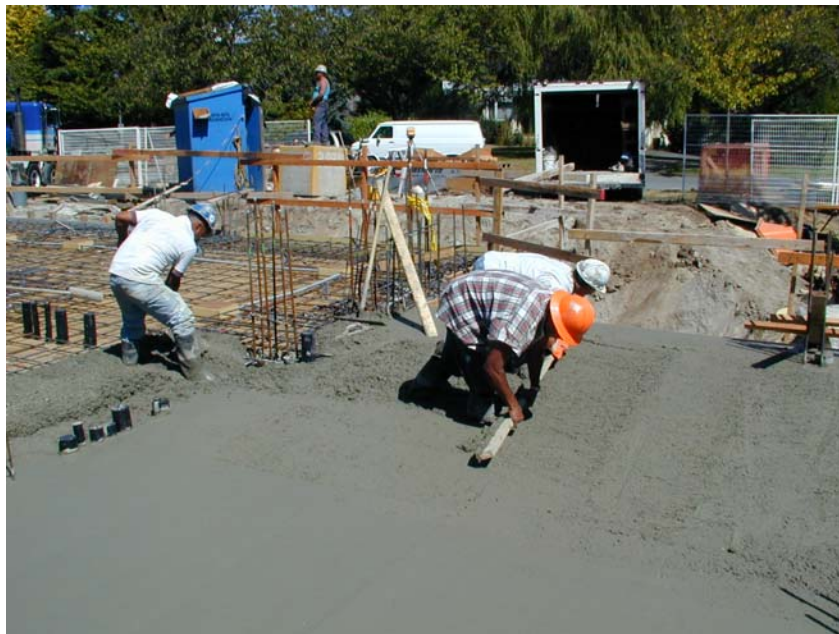
Figure 7: Screeding the Concrete
