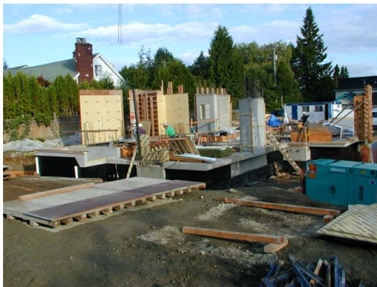
Figure B-4: View during Ground Floor Construction
