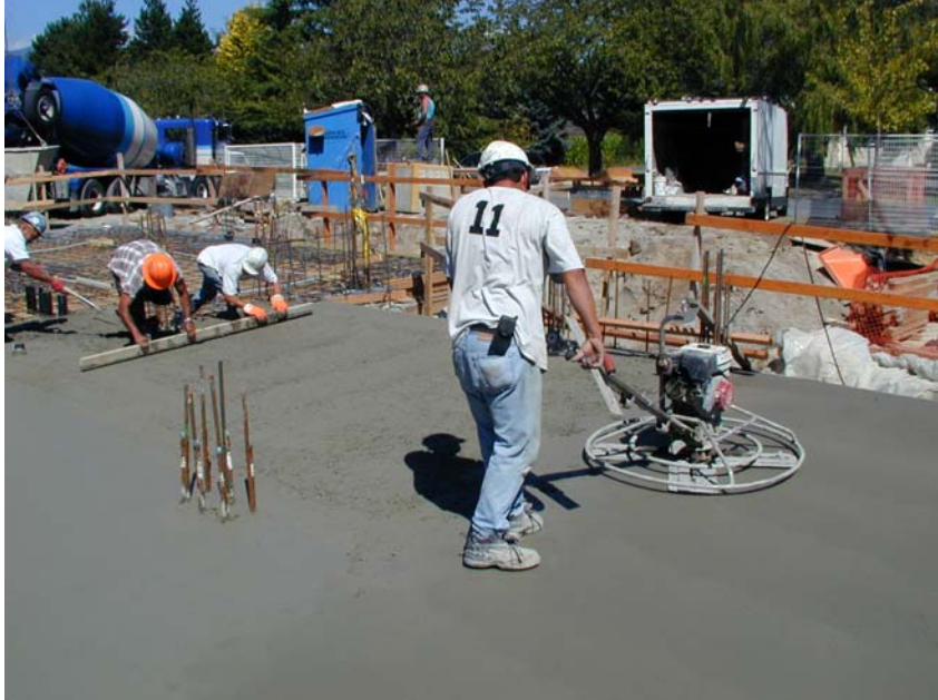
Figure 8: Power Trowel Finishing the Concrete
