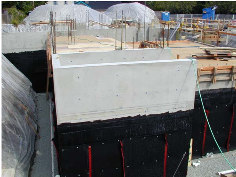
Figure 2: View of Exposed Section of Basement Wall
