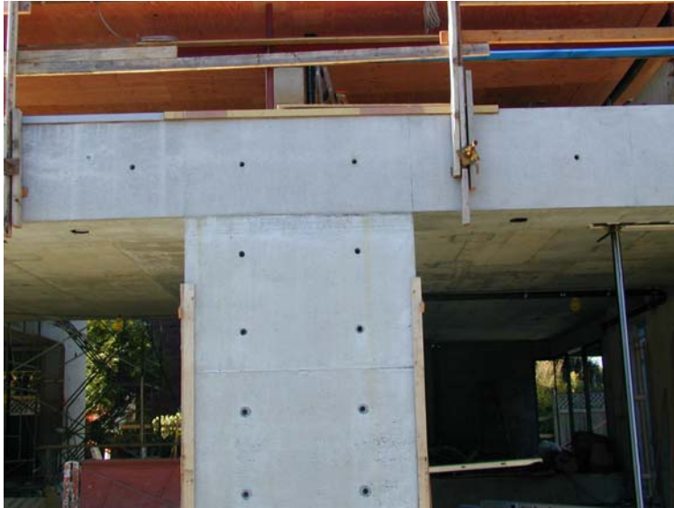
Figure B-3: Close-up of Form Fresh Finish, Wall and Slab Edge Cold Joint
