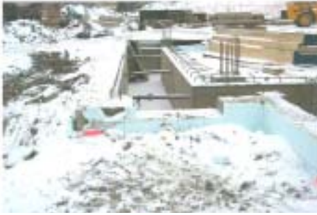
FIGURE F4.1 CONSTRUCTION NOV. 8 TH , 2002
