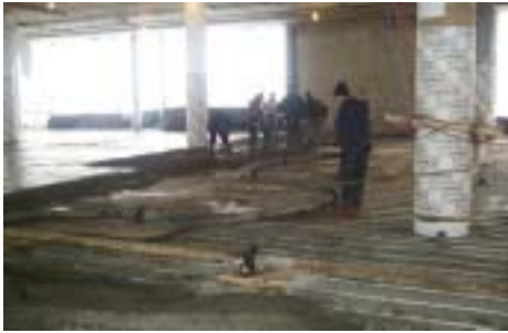
FIGURE F4.4 GROUND FLOOR SLAB POUR (ABOVE RADIANT PIPES)
