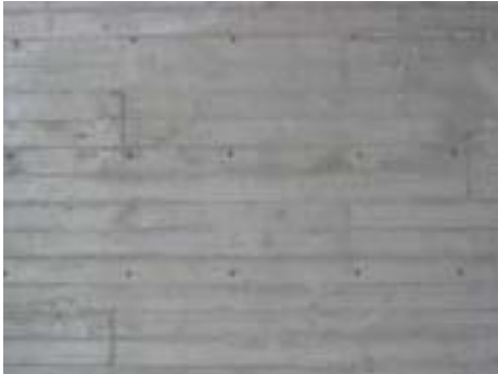
FIGURE F4.5 BOARD FORMED CONCRETE WALL
