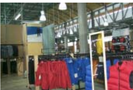
FIGURE F4.7 DULLED SHINE ON TOP OF COLUMNS
