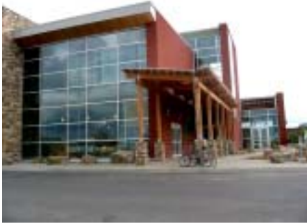
FIGURE F1.1 SALVAGED WOOD IN ENTRANCE CANOPY
