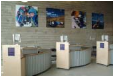
FIGURE F3.5 BOARD FORMED SHEAR WALL BEHIND CASH AREA
