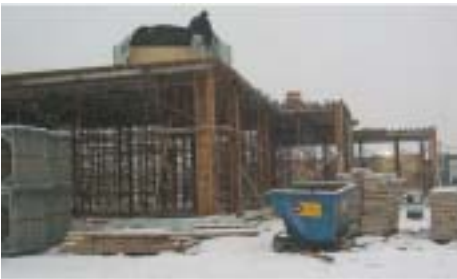
FIGURE F4.2 FORMWORK FOR STRUCTURAL SLAB NOV. 29 TH , 2002
