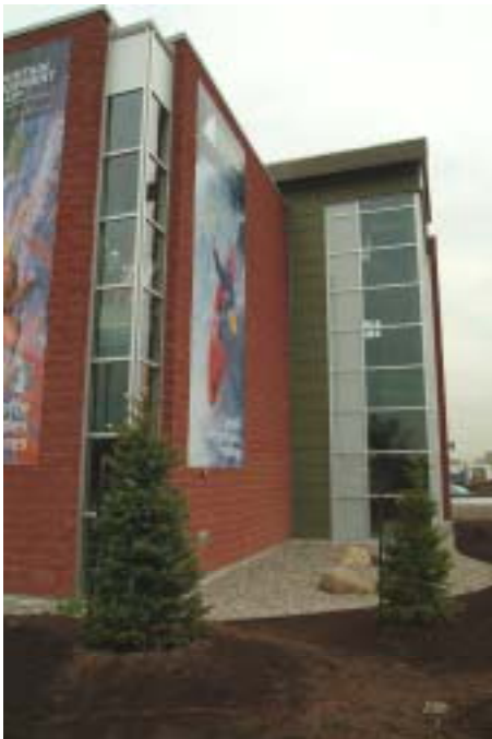
FIGURE F6.1 SOUTHEAST CORNER: GLAZED CORNER BEHIND CLIMBING WALL
