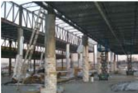
FIGURE F4.6 ROUND COLUMNS WITH LINERS
