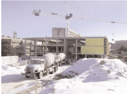
FIGURE 2.4.2a YORK UNIVERSITY COMPUTER SCIENCE BUILDING
