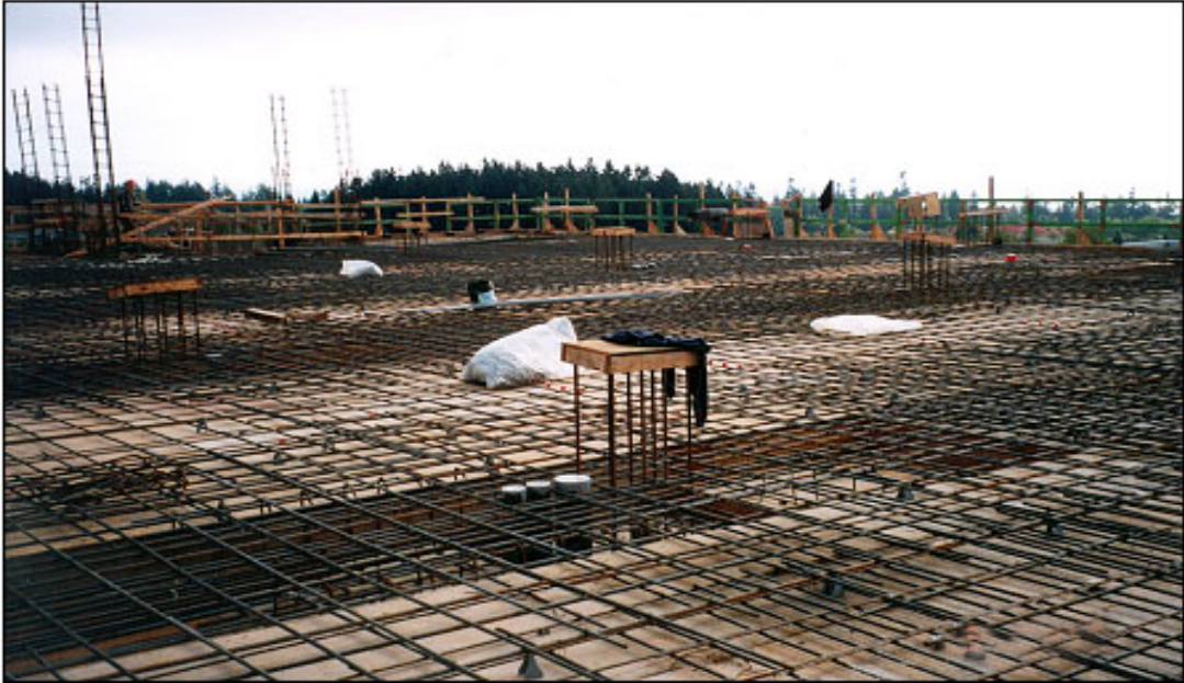
FIGURE 6 TECHNOLOGY ENTERPRISE FACILITY III, UBC Slab Under Construction
