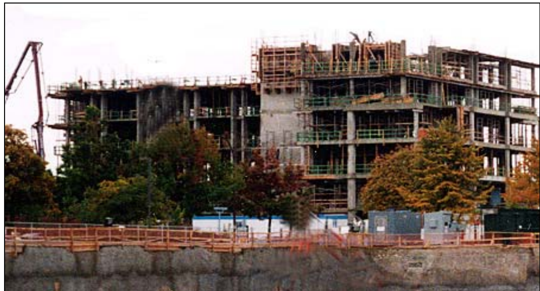
FIGURE 3 TECHNOLOGY ENTERPRISE FACILITY III, UBC East Elevation – Under Construction
