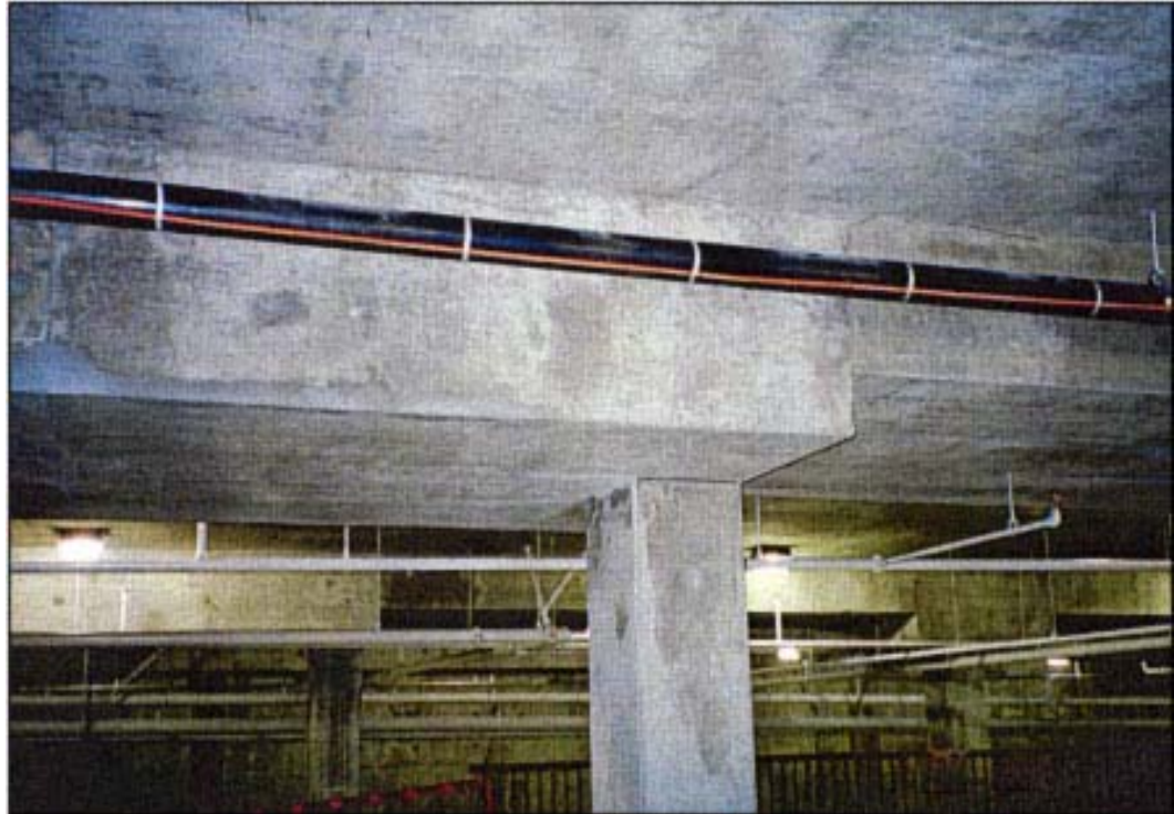
FIGURE 5 TECHNOLOGY ENTERPRISE FACILITY III, UBC Column in Parkade
