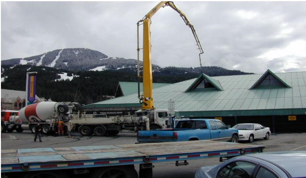
**Figure 2: Pumping Concrete into Building for New Slab on Grade Placement (January 2003)**
