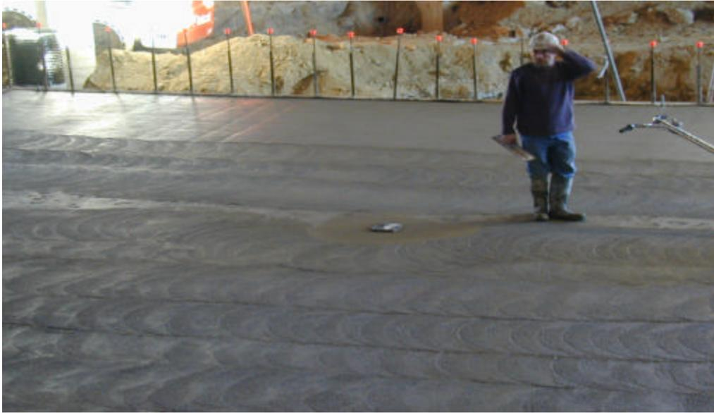
**Figure 3: Finished Slab on Grade Section (35% fly ash content)**
