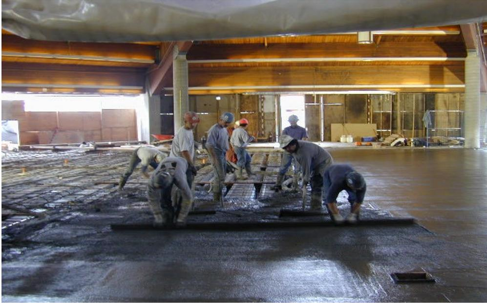
**Figure 1: Concrete Finishing Crew on the Suspended ComFlor Deck System (40% fly ash content)**
