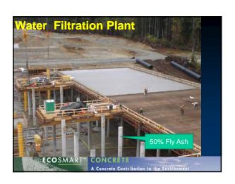
Fly ash is the by-product of coal-fired power plant
