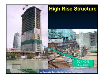
Fly ash improves concrete durability and resistance to sea salt and sulfate.
