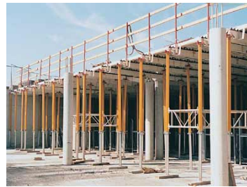
PROPRIETARY FORM SYSTEM
