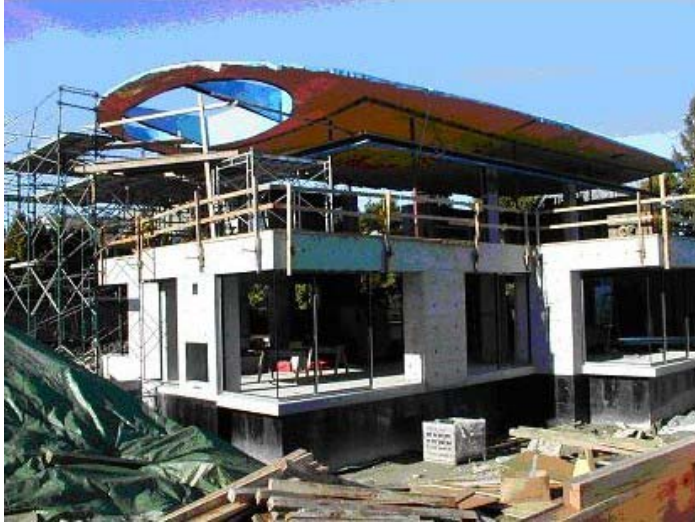
Figure 1 The Lo House under construction.
