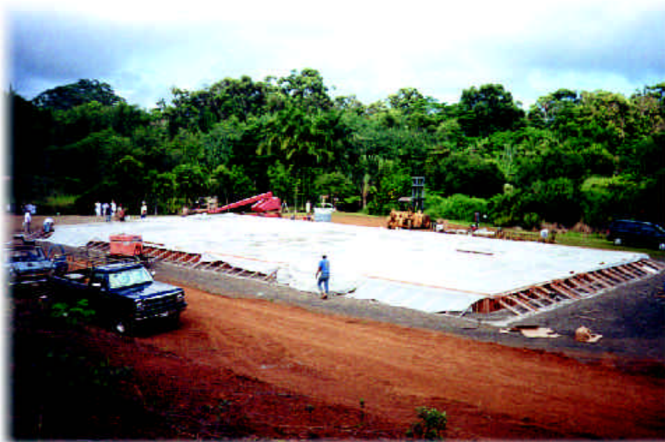
Fig. 3 — Burlap covered with visqueen sheet to prevent drying.
