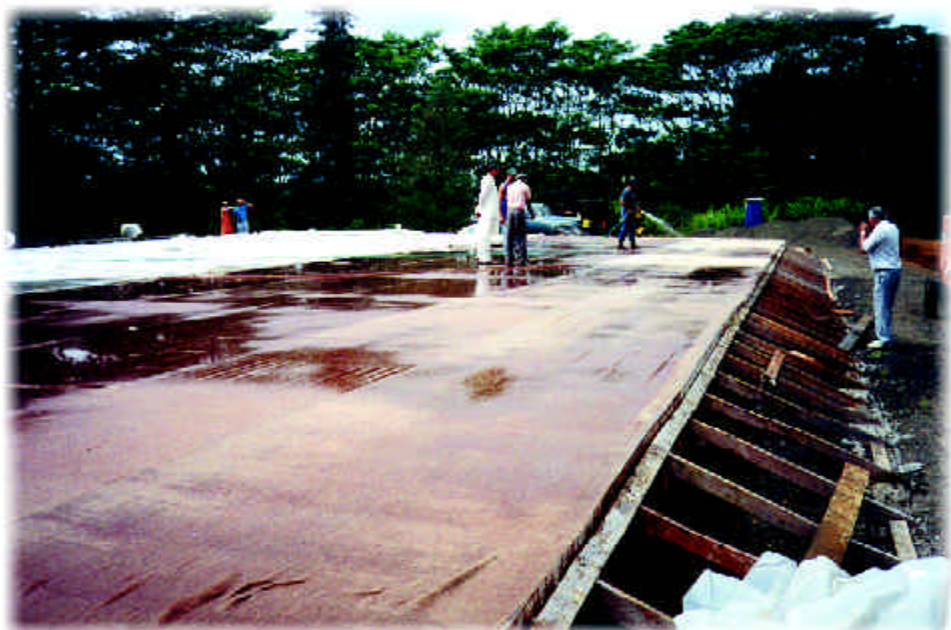
Fig. 2 — Application of burlap and moisture.
