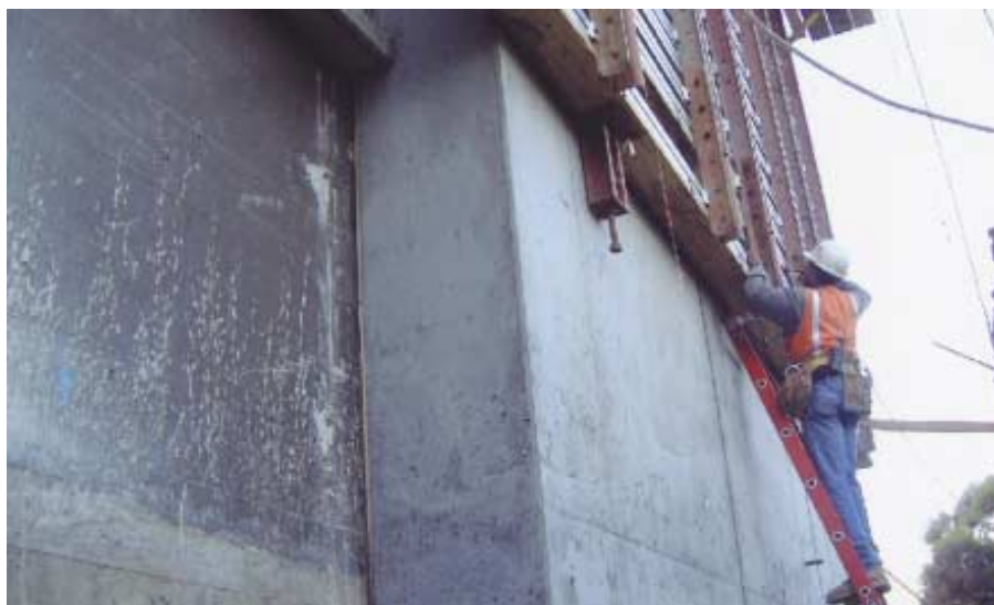
Fig. 4: New shearwalls with forms being removed after 14 days of curing
