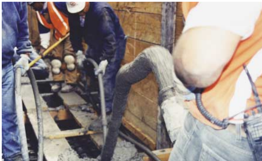
Fig. 3: Workers placing the easily-flowing HVFA concrete into the belt foundation
